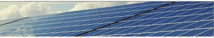
PV panels consist of solar cells that convert light directly into electricity. Solar cells produce direct current (DC) electricity from light, which can be used to power equipment or to recharge a battery. The majority of PV modules are used for grid-connected power generation. In this case an inverter is required to convert DC to alternating current (AC). For Aqaba, a minimum solar yield of 1,350 kWh/kWp needs to be proven by a dynamic simulation tool (e.g. PV Sol, PV Syst, Polysun).
